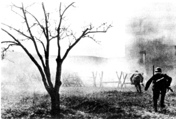
On June 17, 1942, Fort Maxim Gorki I, the main Soviet defensive work in the northern sector, was taken by storm after a heavy bombardment. Here German Sturmpioniere (combat engineers) attack a bunker in this strongest and most modern of the Sevastopol forts. German Official
