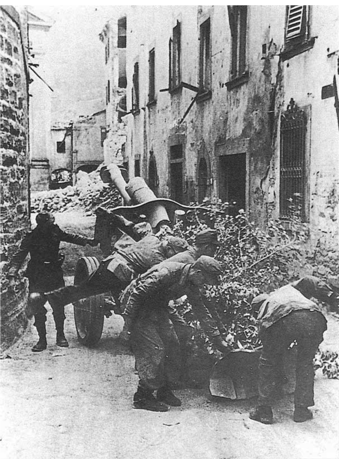
Left: German gunners manhandle their 105mm leichte Feldhaubitze 18 (Mundungbremse) artillery piece into position on the streets of Cherbourg, June 1944. The gun is a refinement of the normal 105mm leFH 18, with a modified recoil system and muzzle brake to take a stronger charge in the shell.
