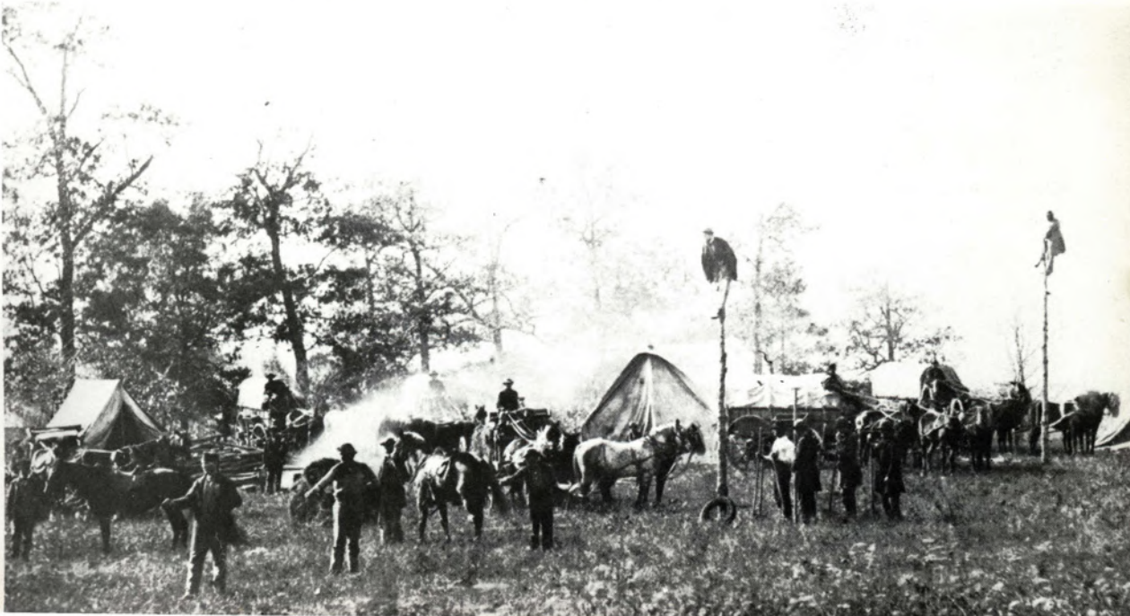
BELOW: Men of the US Signal Corps erecting telegraph poles. Photographed by Timothy O'Sullivan in 1864
