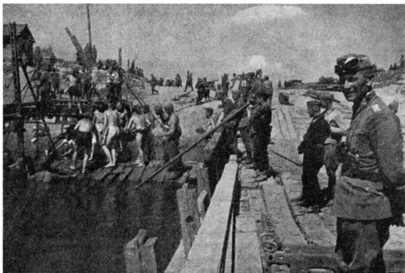
Fig. 12. Bridge building over the Dnieper near Kopys
