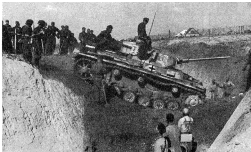
Fig. 17. An anti-tank ditch in the Stalin line
