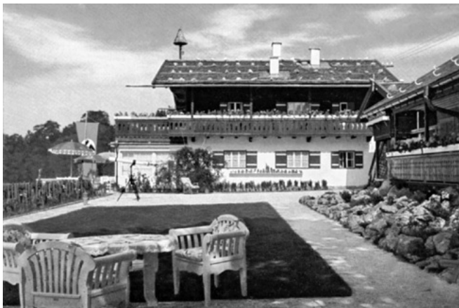
The Berghof after the 1935–1936 renovations (Illustration Credit 8.2)
