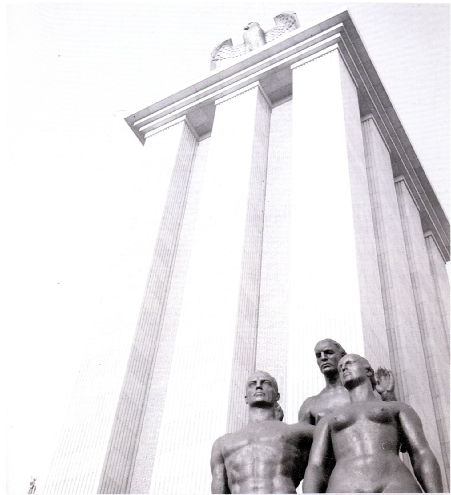
GERMAN PAVILION AT THE UNIVERSAL FAIR IN PARIS IN 1937 The area allocated to the German pavilion was right in front of the Soviet Union's. Speer got to know in advance what the Russian pavilion was to look like, so he designed one for Germany that in size equalled if not surpassed that of the Reich's main ideological adversary.
