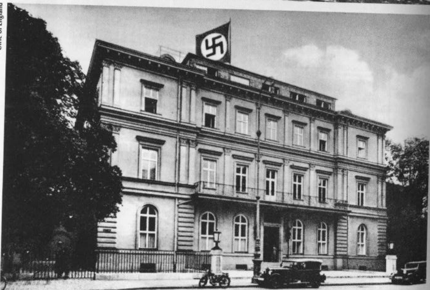
Two views of the Braune Haus taken from the right and the left. The new entrance by Troost can be seen along with the new front flanked by pillars bearing lights.
