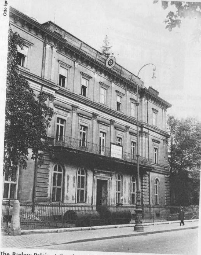
The Barlow-Palais at the time of purchase by the NSDAP in 1930. The white notice above the door states that this building has been purchased by the NSDAP. On the roof a temporary round swastika sign was placed bearing the dedication "DEM ERWACHENDEN DEUTSCHLAND."
