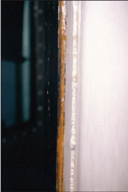
Fig. 101: Closeup of rubber seal around gas chamber door, also covered in Vaseline when in use.
