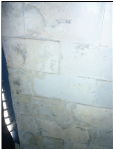
Ill. 50: Newly added tiles, or rather, fake tiles, around the introduction chutes.
