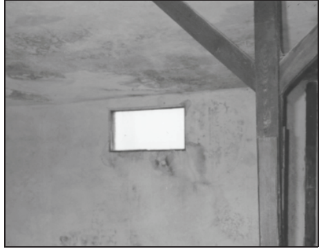
Fig. 30: Window in Chamber IV of Building no. 41, Majdanek camp; until 2005 claimed to have been a homicidal gas chamber, but now admitted to have been a mere delousing chamber. © C. Mattogno
