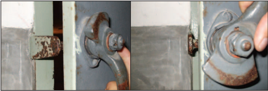
Ill. 59a & b: The doors to the alleged gas chamber at Dachau cannot be closed nowadays: a missing closing mechanisms and blocking steel pins welded to the frame prevent this.
