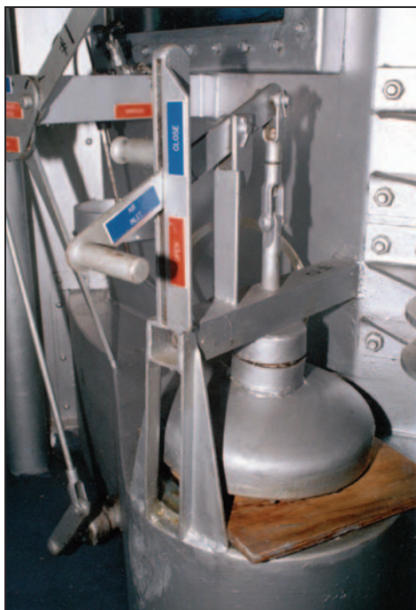
Fig. 95: Closeup of fresh-air intake of gas chamber.
