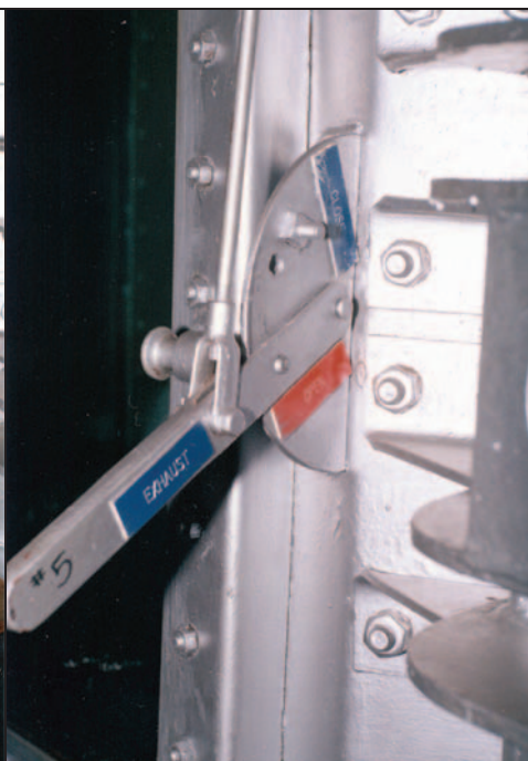
Fig. 96: Closeup of lever used to open and close exhaust stack.
