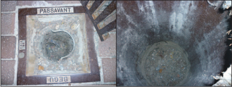
III. 60a & b: One of the six floor drains inside the alleged gas chamber at Dachau. Left: grate removed, sieve in place; right: sieve removed; the exit drain pipe can be seen at the drain's bottom (top-most spot of the bottom).
