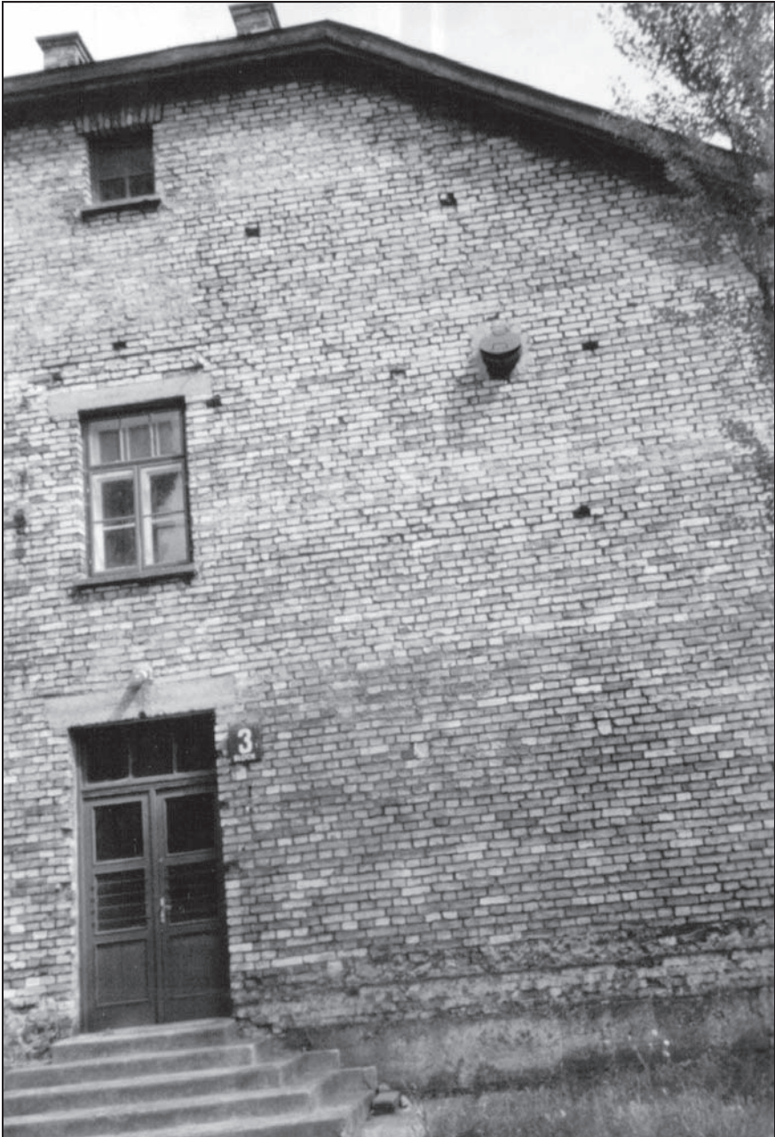
3. Auschwitz, Block 3. Round opening covered by a metal lid, which housed the ventilator for the gas disinfestation chamber located on the second floor of the Block. July 1992, © Carlo Mattogno.
