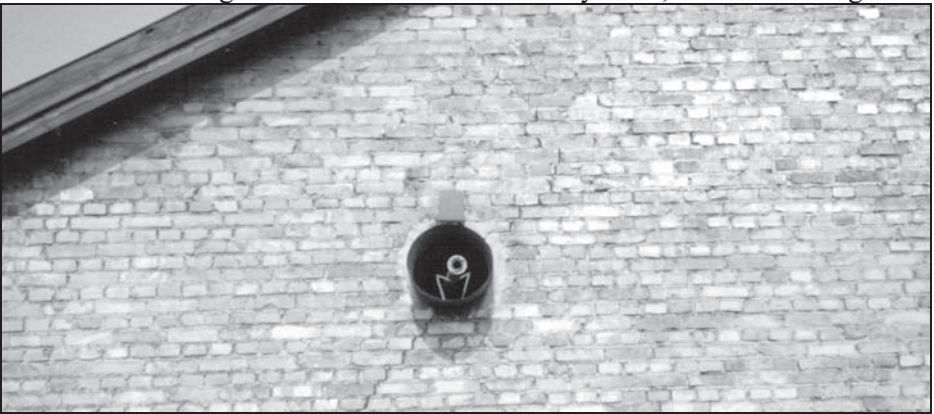
2. Birkenau, BW 5b. One of the two round openings for placement of ventilators in the outside wall of the gas disinfestation chamber. Above the sheet metal tube one can see, attached to it by means of a hinge, a metal plate to which the lid of the tube was welded. July 1992, © Carlo Mattogno.
