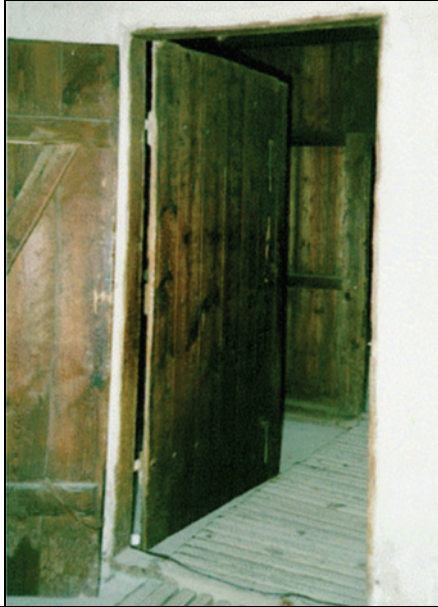
Photograph XVII: Barrack 41, gas chamber, north door. The inside of the door is marked by the typical discolorations that are also visible on the outside of the south door (Photograph XVIa); hooks for the latches are missing from the door frame, unlike on the frame of the south door (Photograph XVI). (© Carlo Mattogno)
