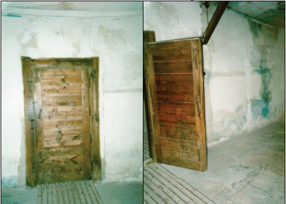
Photograph XVI, XVIa: Barrack 41, gas chamber, south door. In the left part of the door there are three latches which are inserted into the three corresponding hooks on the door frame via handles operated from the other side of the door (Photograph XVIa). (© Carlo Mattogno)
