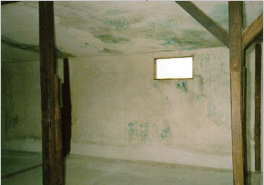
Photograph XX: Barrack 41, gas chamber, window in the east wall. (© C. Mattogno)
