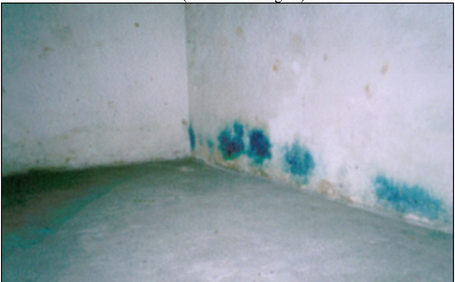
Photograph XIV: Disinfestation facility, Barrack 41, Chamber II, west wall. (© Carlo Mattogno.)
