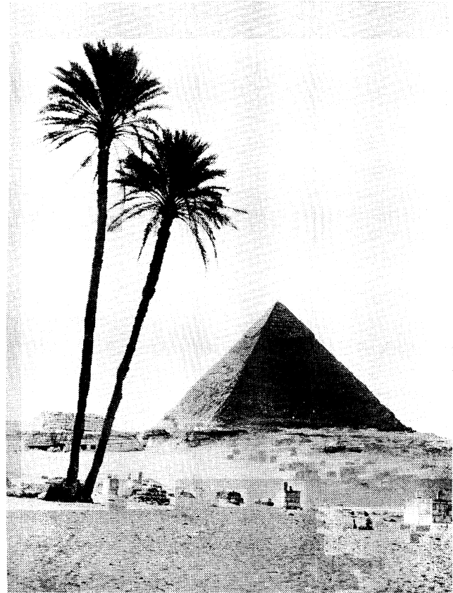
The pyramid of king Khafre (Kha-f-Ra). This is the second-largest of the three great pyramids of Giza, which were built during the IVth dynasty, between 2686 and 2613 B.C. It has a perpendicular height of 447-1/2 feet. At the top a fragment remains of the original coating of limestone and unpolished granite slabs.
