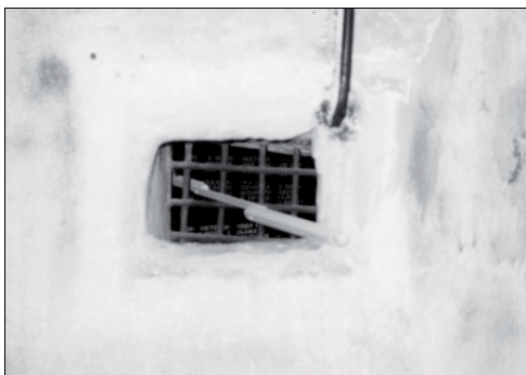
Illustration 4: Unsealed opening with nothing more than a grate links Chamber I to the small attached room, hut 41, concentration camp Majdanek (cf. map, illustration 1). © C. Mattogno
