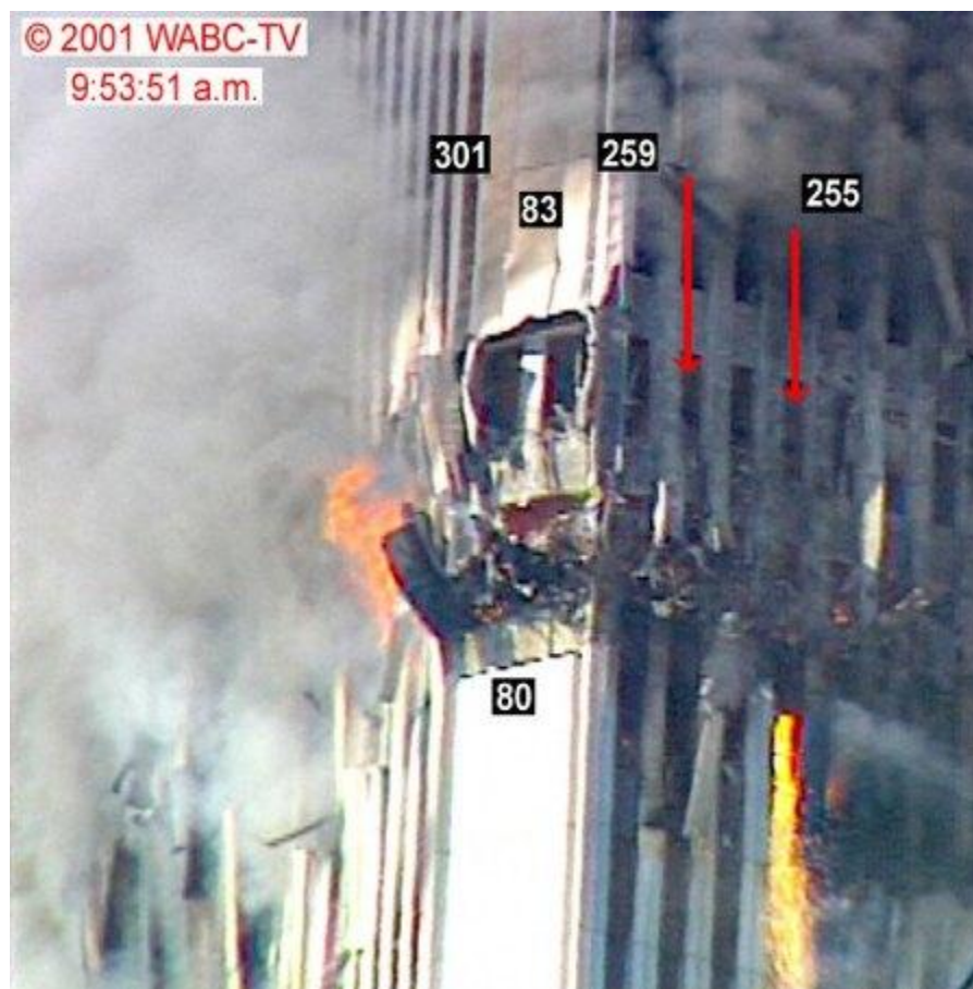
Molten iron pours out of South Tower about one minute before the tower disintegrated.
