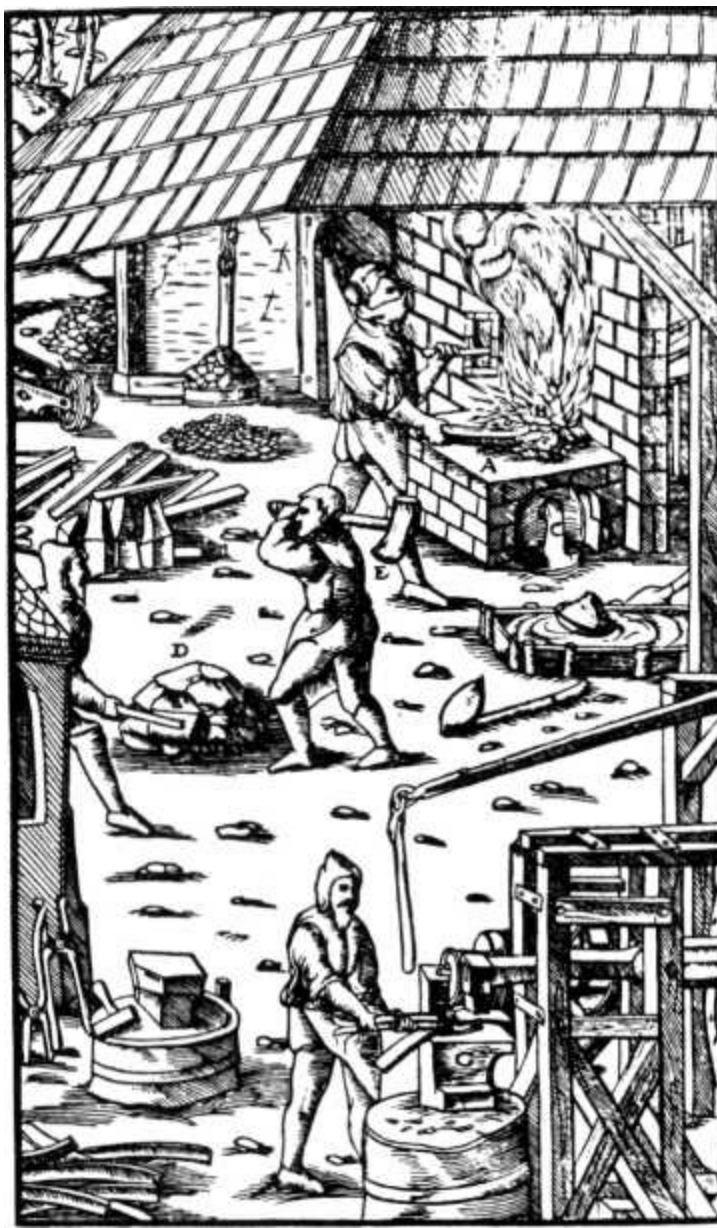
Figure 17. Iron-smelting furnace and forge, mid-sixteenth century.
