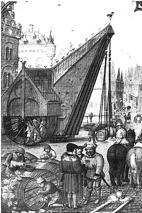
The crane at Bruges, in the middle ages: a massive wooden construction with a huge wheel operated by three men. (Bayerisches Staatsbibliothek, Munich.)
