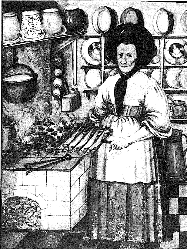
Cooking without bending down: the German fireplace with raised hearth (1663). From the Mendelsche Bruderbücher ( Books of the Companions of the Mendel Foundation ), Stadtbibliothek Nurnberg, Nuremberg. (Photo Armin Schmidt.)
