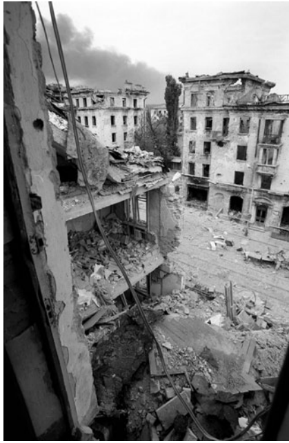
Plate 24. Grozny, the capital city of the republic of Chechnya, in ruins after battles between the Russian armed forces and nationalist resisters, 1996.
