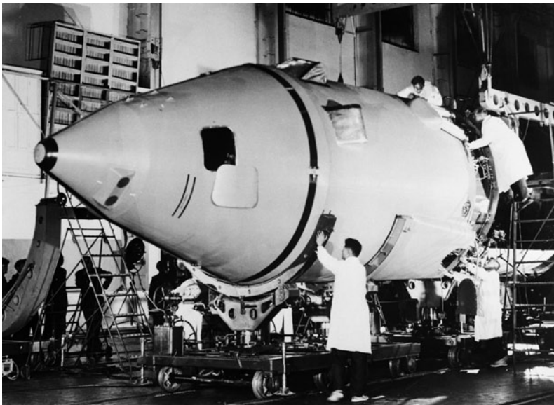
Plate 18. Soviet space capsule Vostok being assembled in 1965 by a group of Soviet technicians; photograph released by an official Soviet source in connection with the USSR Economic Achievement Exhibition in Moscow.
