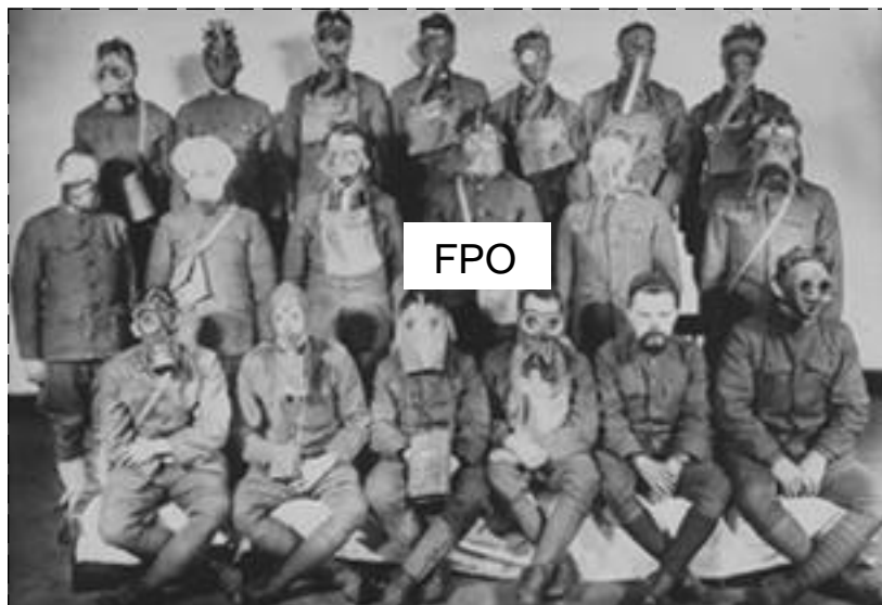
Fig. 2-5. A potpourri of World War I-vintage protective masks. This extraordinary photograph gives some indication of the great effort made by the warring parties to develop an effective and practical (and frequently unsuccessful) defense against the chemical warfare threat. Top row, left to right: U.S. Navy Mark I mask; U.S. Navy Mark II mask; U.S. CE mask; U.S. RFK mask; U.S. AT mask; U.S. KT mask; U.S. model 1919 mask. Middle row, left to right: British Black Veil mask; British PH helmet; British BR mask; French M2 mask; French artillery mask; French ARS mask. Bottom row, left to right: German mask; Russian mask; Italian mask; British Motor Corps mask; U.S. Rear Area mask; U.S. Connell mask. Photograph: Chemical and Biological Defense Command Historical Research and Response Team, Aberdeen Proving Ground, Md.
