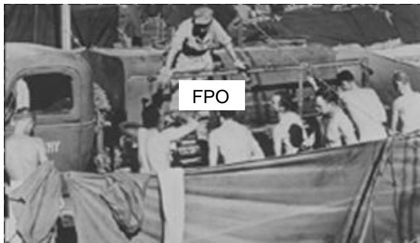
Fig. 2-39. The 400-gal decontaminating apparatus was also used to provide water showers for the troops on Iwo Jima. Like the actual weapons, all the associated paraphernalia of chemical warfare had to go with the deployed combat forces. Useful alternative work was found for decontamination apparatuses, however, in contrast to the bombs shown in Figure 2-34. Photograph: Chemical and Biological Defense Command Historical Research and Response Team, Aberdeen Proving Ground, Md.
