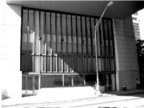
The site of the National Pencil Company (37 S. Forsyth St.) where Mary Phagan was murdered, now the Sem Nunn Federal Center.
