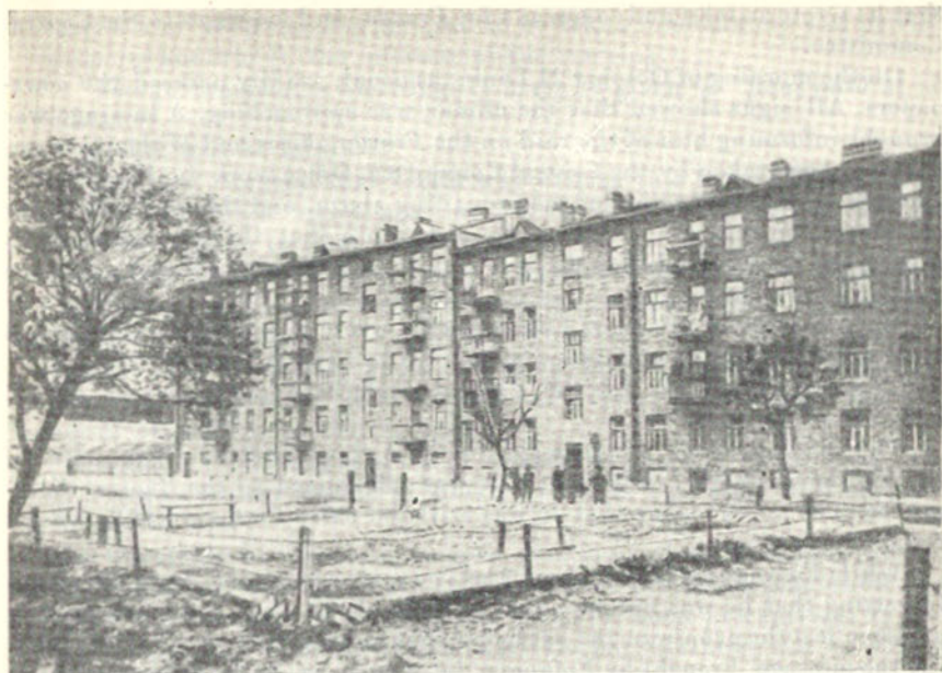
House No. 92/1 on the corner of Sampsonievsky Prospect and Serdobolskaya Street in Petrograd where in Flat No. 42 Lenin lived in hiding after his return from Finland up to October 25 (November 7) 1917.
