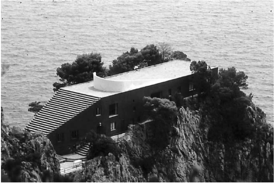
Figure 6 Adalberto Libera's highly modernist house built for Curzio Malaparte on Capri.
