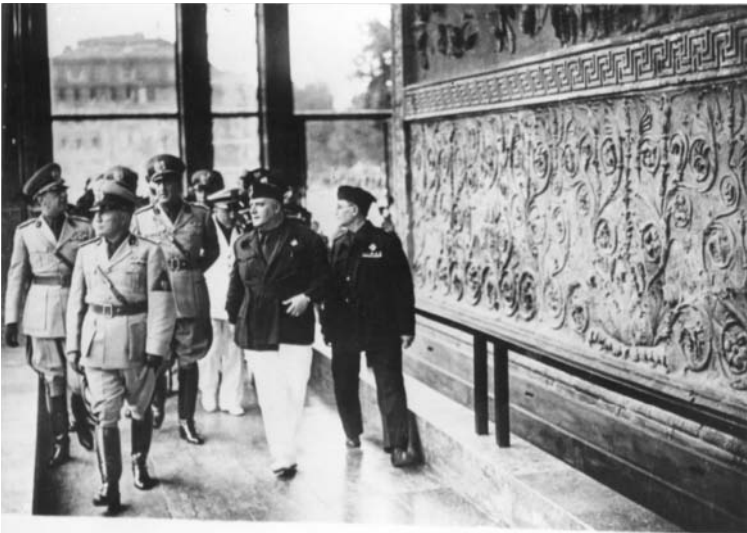
Figure 5: Mussolini opening the building to house the Ara Pacis on 23 September 1938. Note the classical swastikas on the frieze. My thanks to Orietta Rossini for supplying this photo and giving me permission to use it.
