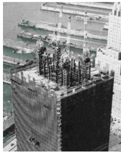
WTC 1 during construction.
