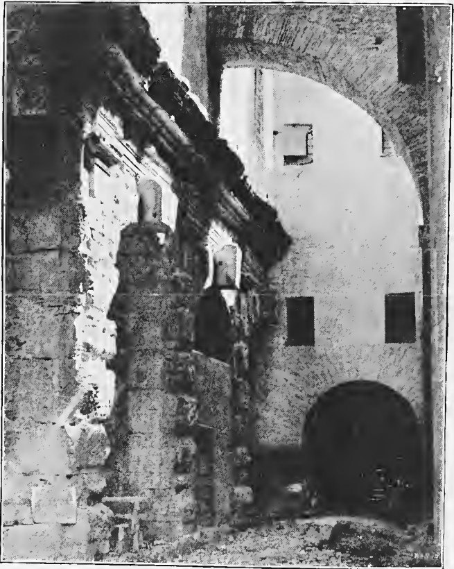
Fig 133. — The Substructures of the Claudium, West Side.
