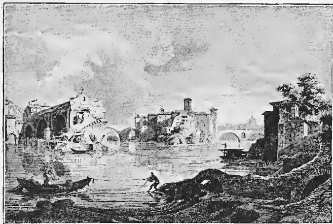
Fig. 8. — The Æmilian, Fabrician, Cestian Bridges, and the Island in the Tiber.
