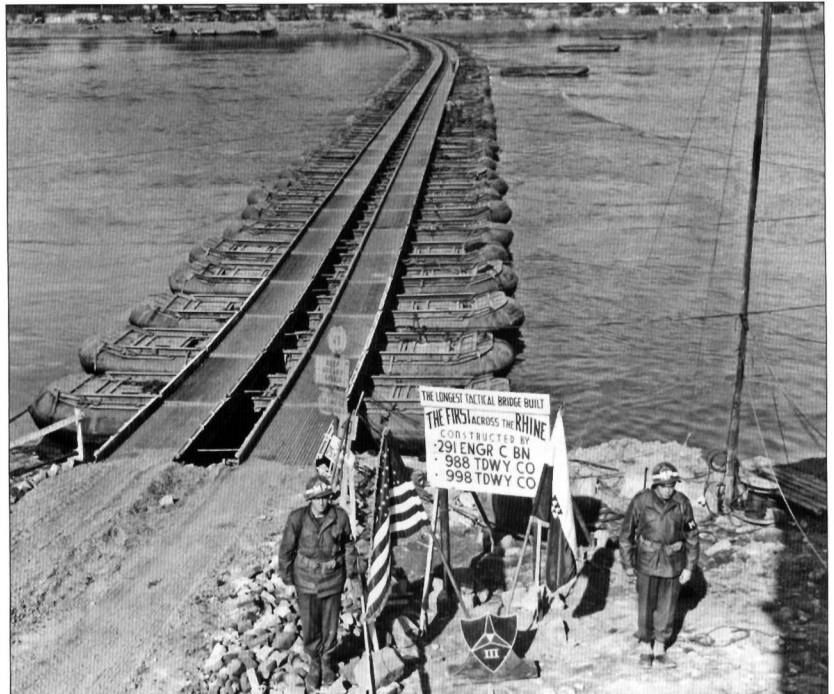
The first of the tactical bridges across the Rhine near the Ludendorff Bridge was a treadway bridge constructed by the 291st Engineer Combat Battalion completed early on the morning of May 11. (NARA)
