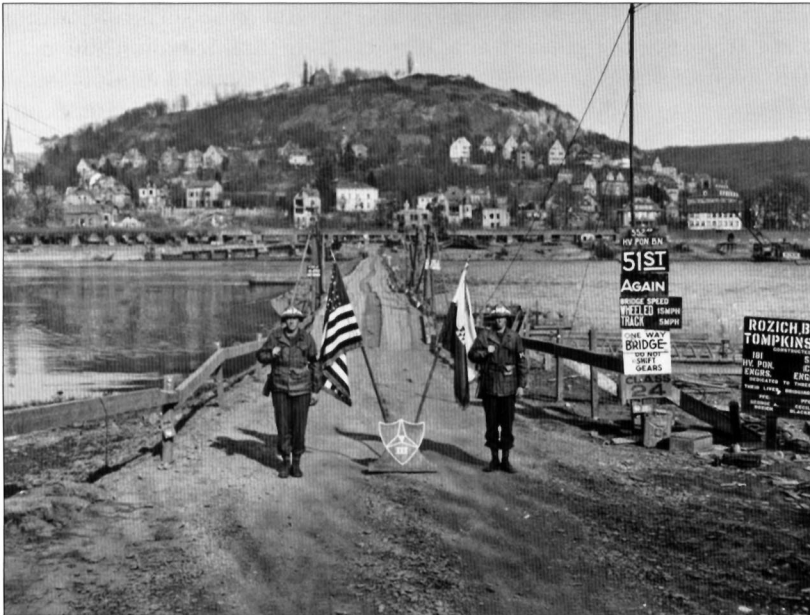
A pontoon bridge was constructed south of the Ludendorff Bridge between Kripp on the west bank and Linz by the 51st Engineer Combat Battalion late on March 11. (NARA)
