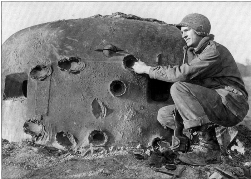
The First Army exited the fortified Westwall defenses during the February fighting. Here a GI from the 76th Division looks at the damage inflicted on an armored cupola overlooking the Sauer River on February 16, 1945. (NARA)
