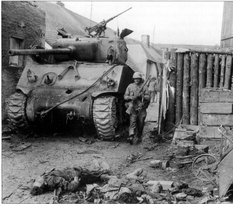
Operation Undertone was aimed at breaking through the German fortified border defenses to close on the lower Rhine. Here, a GI of the 94th Division walks through a gap in a roadblock in Lampaden and past an M4A3 (76mm) of the 778th Tank Battalion that has been knocked out by two gun penetrations through the transmission cover during the fighting for the Saarbrücken bridgehead on March 9, 1945. (NARA)
