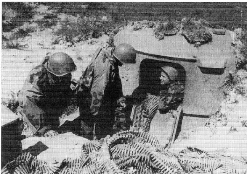
A Soviet scout platoon inspects a German pillbox, typical of the defences approaching Orsha. The Germans made extensive use of pre-fabricated steel pillboxes on the Eastern Front. These were actually intended for incorporation into poured-concrete fortifications, but were sometimes used as parts of earthworks, as seen here. (Sovfoto)
