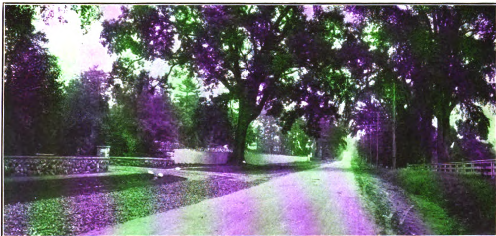
BITUMEN MIXED WITH MACADAM TO MAKE A FINE ROAD IN NEW JERSEY
