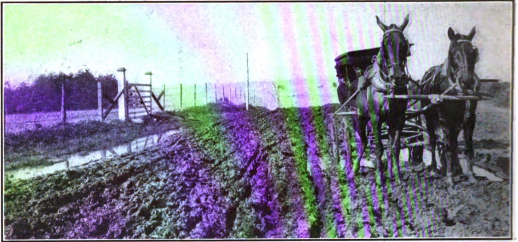
A ROAD IN SPOTTSYLVANIA COUNTY, VA., AS IT LOOKED IN 1910 TYPICAL OF THE ORDINARY COUNTRY ROAD AFTER A HEAVY RAIN, CUT INTO RUTS AND SINKS
