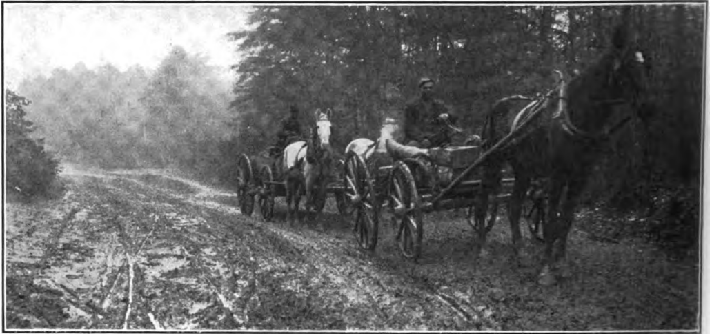
A LOAD OF LUMBER ON A BAD ROAD
