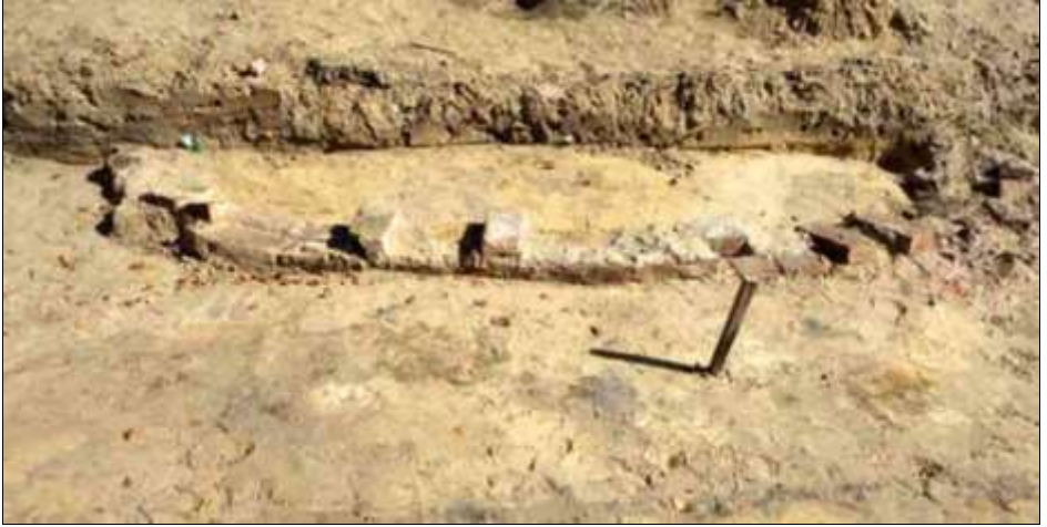
Document 46: Remnants of the foundation walls of the alleged gas chambers at Sobibór. Alleged Gas Chamber No. 3. Seen from west to east. Semi-circular side wall. Image in the public domain.
