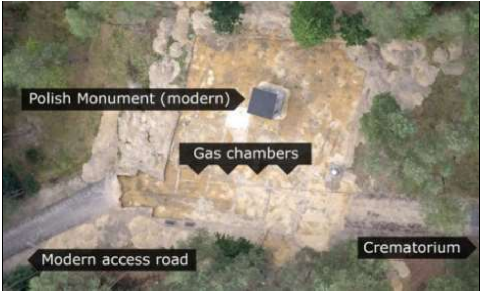
Document 43, 43a: Remnants of the foundation walls of the alleged gas chambers at Sobibór. Hecking, p. 6. I added explanatory letters and numbers to Document 43a (see text).
