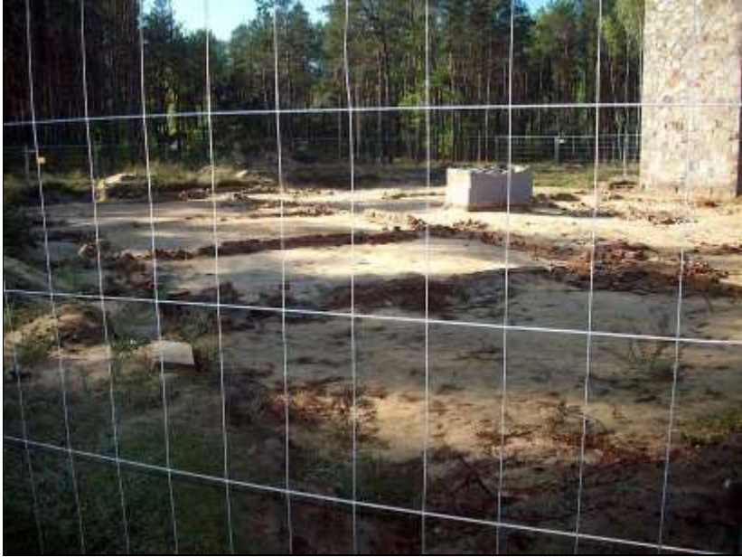
Document 56: Remnants of the foundation walls of the alleged gas chambers at Sobibór (2015). Seen from northeast to southwest. © Carlo Mattogno.
