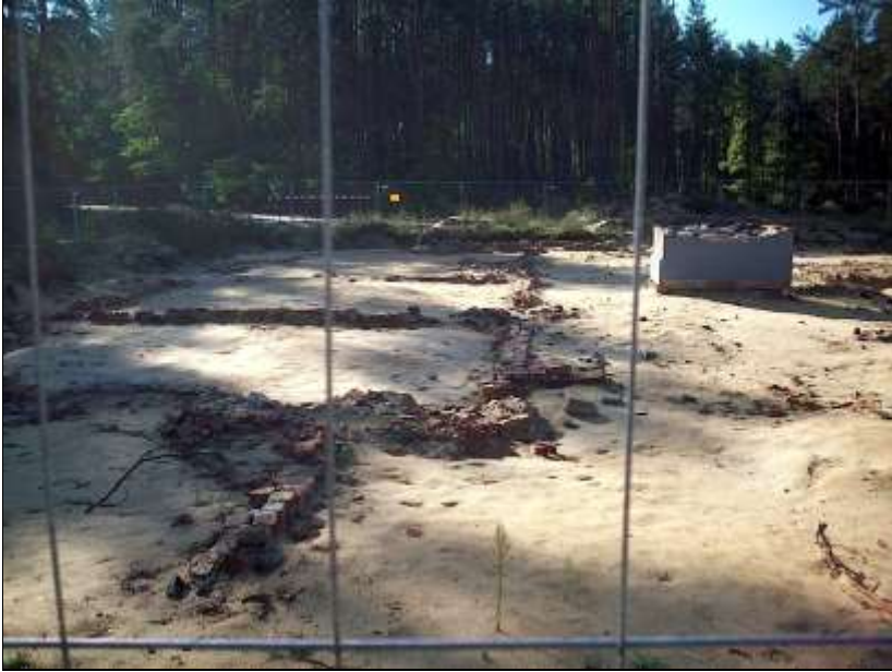
Document 54: Remnants of the foundation walls of the alleged gas chambers at Sobibór (2015). Seen from north to south. © Carlo Mattogno.
