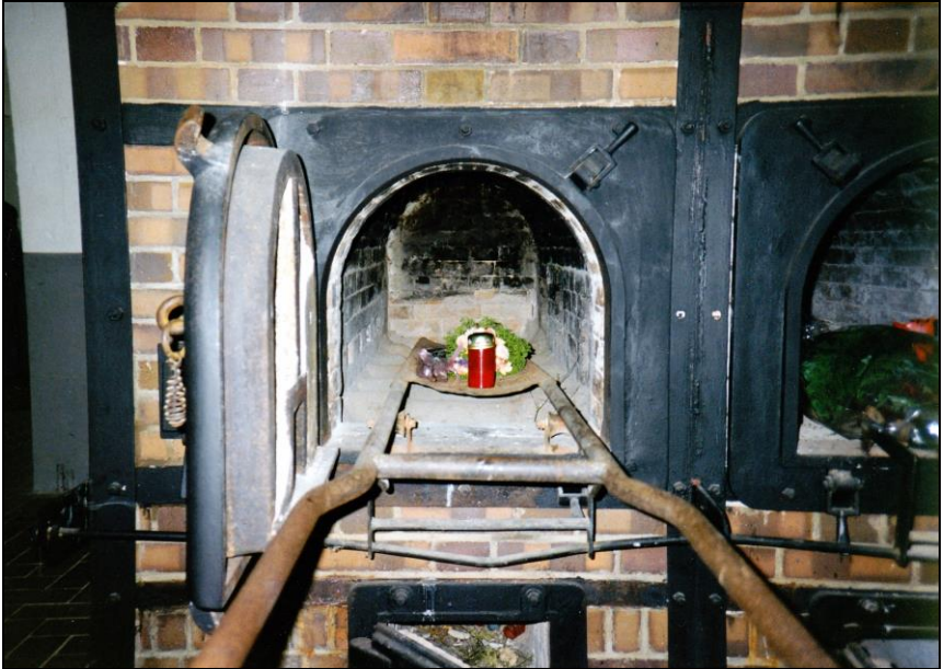
Document 44: Crematorium of Mauthausen. Topf coke-fired double-muffle furnace, Auschwitz Type. Loading system of furnace: fixation shaft, mobile roller system and corpse stretcher. Viewed from above. © Carlo Mattogno.
