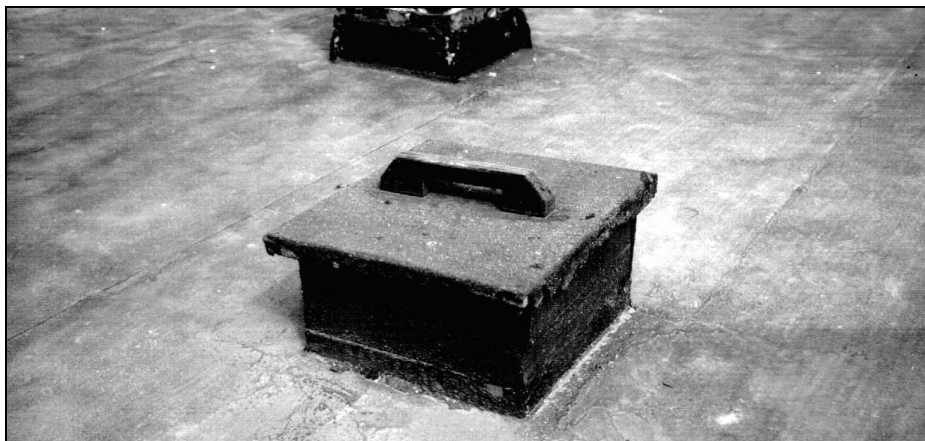
Document 24: Photo of the roof of the morgue. One of the four shafts constructed by the Poles after the war. © Carlo Mattogno
