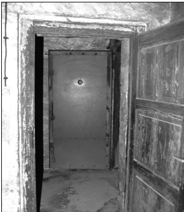
Document 30: Auschwitz, old crematorium, gas-tight door of the air-raid shelter (rear entry); at the right: wooden door of the vestibule. © Fredrick Töben 1997
