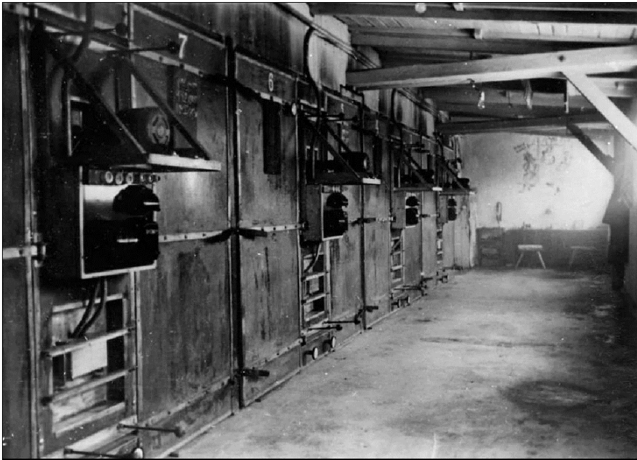
Figure 35: Four hot-air disinfestation chambers in the shower and delousing building of the Gypsy Camp, Birkenau (1943; Pressac 1989, p. 63).
