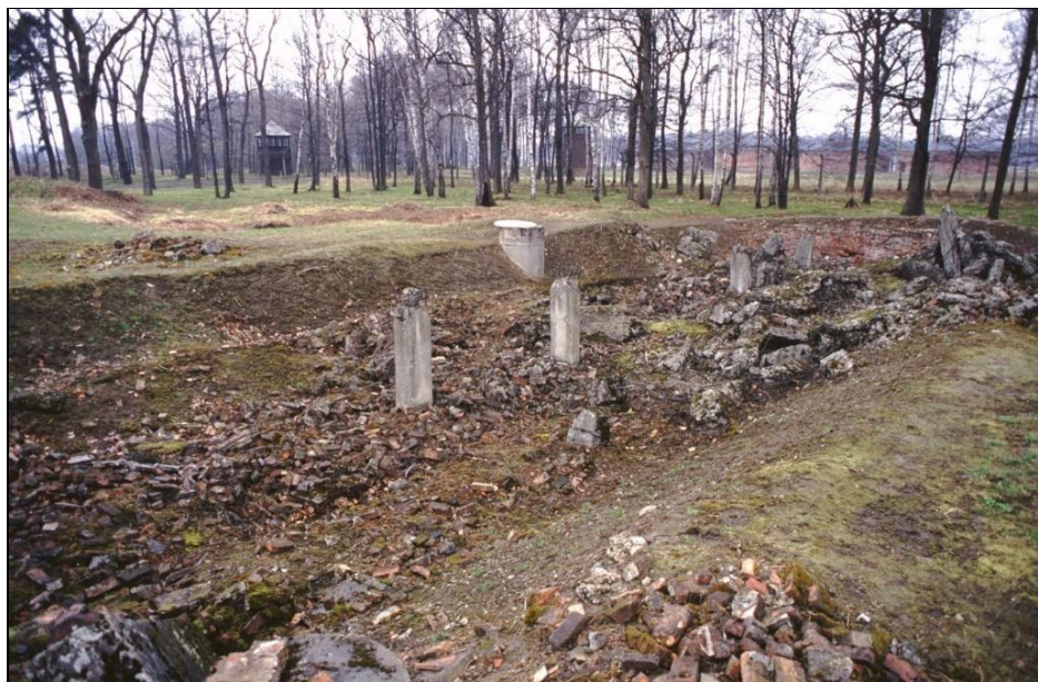
Figure 70: Morgue #1 of Crematorium III, with its roof utterly demolished (February 1997.).
