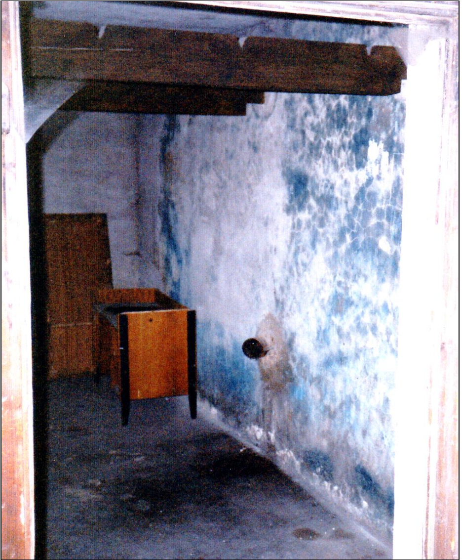
Figure 159: Disinfestation wing of Building 5a, eastern internal wall seen from the south, not quite as intensely stained as external walls (Room 1 in Figure 40, seen from the south). (© C. Mattogno 1991)
