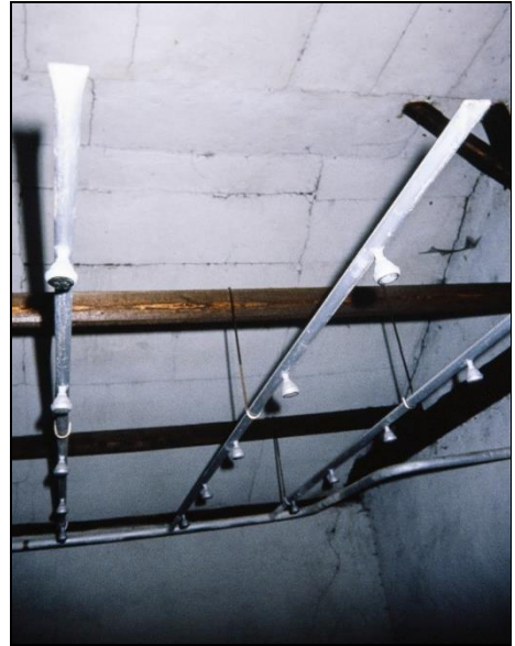
Figure 43: Water-pipe system with shower heads in the disinfestation wing of building BW 5b. These water pipes have no connection; they terminate in the ventilation outlets. See Figure 42.
