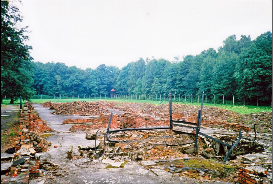
Figure 107: Ruins of Crematorium V. In the foreground the wrought-iron frame of the Topf eight-muffle furnace (© 1997 Mattogno 2015e, Vol. 3, p. 144)
