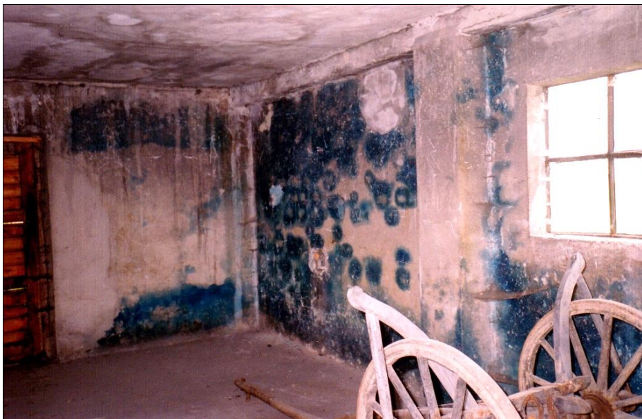
Figure 155: Disinfestation wing of Building 5a, with the southern external wall on the left and the western wall on the right (Room 3 in Figure 40). (© C. Mattogno 1992)
