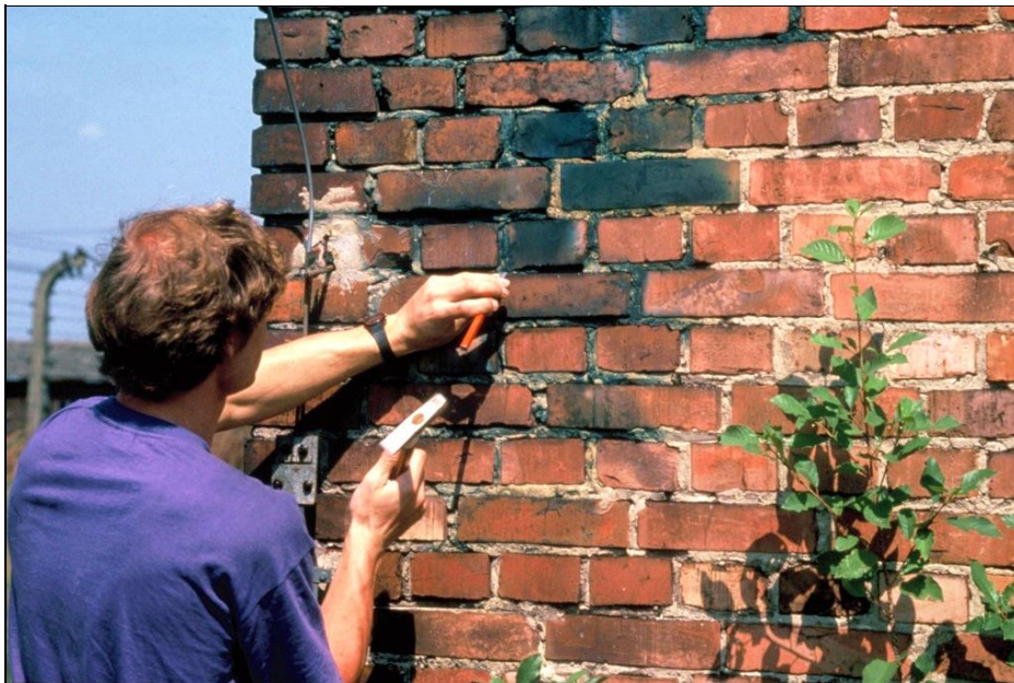
Figure 145: The outside of the southern external wall of hydrogen-cyanide-delousing wing of Building 5a in August 1991 with the author. Small amounts of cyanide which diffused through the walls are discoloring them at places still today. 50 years of the most detrimental environmental influences did not efface this.
