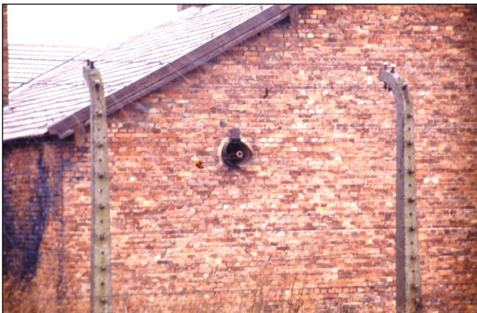
Figure 42: Ventilation outlets from the disinfestation wing of Building 5b, without equipment today. The ends of the water pipes are visible inside; see also Figure 43.
