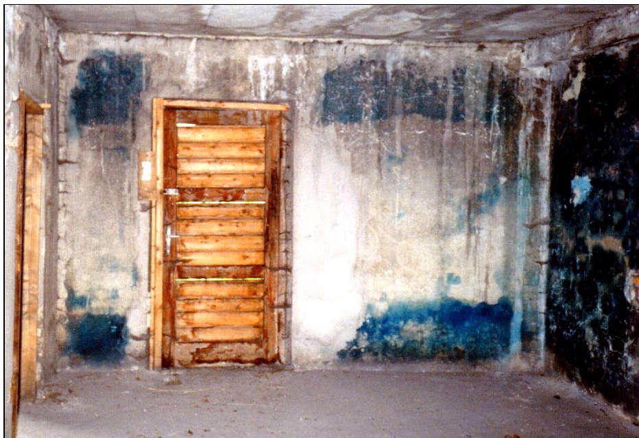
Figure 154: Disinfestation wing of Building 5a, with the southern external wall ahead and the western wall at the right (Room 3 in Figure 40). (© C. Mattogno 1992)
