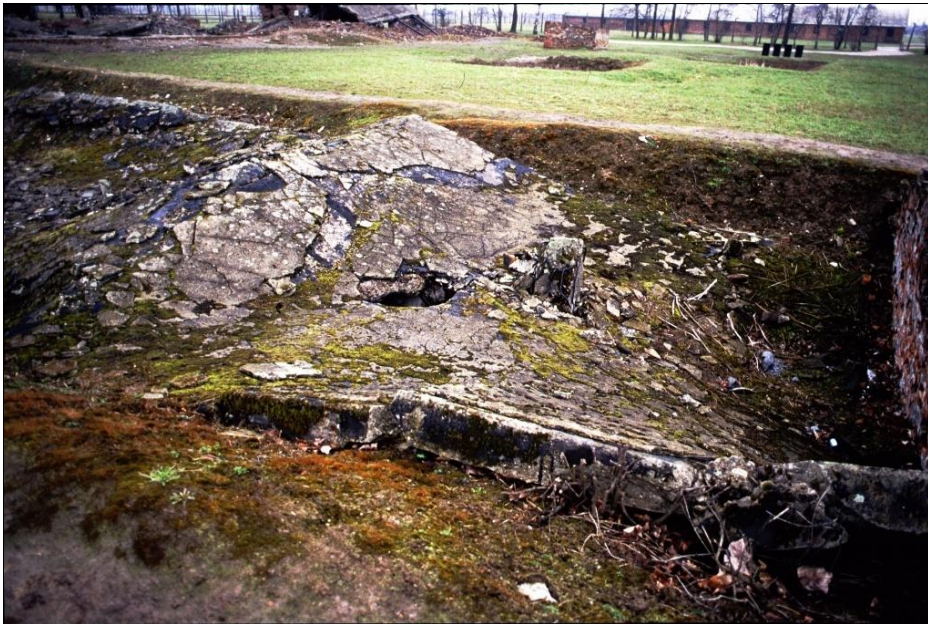
Figure 66: Morgue #1 of Crematorium II in Birkenau, collapsed roof, somewhat-intact rear section still accessible. Center: The last of the seven concrete pillars poking through the roof. A meter or so to the left: a hole chopped through the roof to gain access to the area below (see Figure 84, p. 139). (February 1997)
