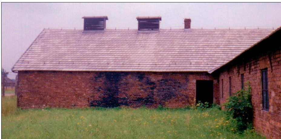
Figure 164: Disinfestation wing of Building 5a, northern wall, with intense staining. (© C. Mattogno 1992)
