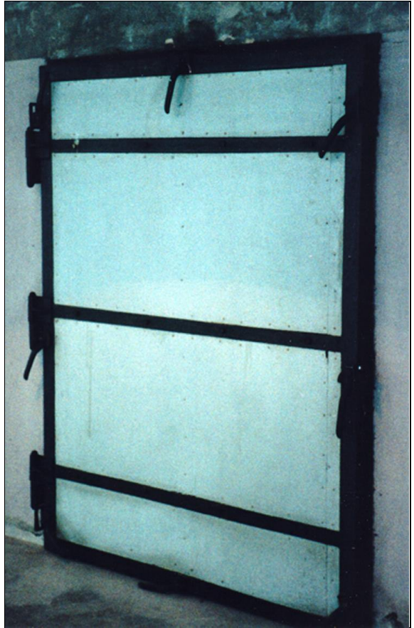
Figure 73: Gastight, escape-proof steel-frame door to one of the Degesch circulation delousing chambers at the Buchenwald Camp. (© C. Mattogno)
